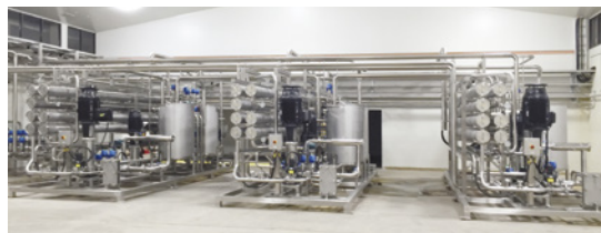
The water recovered from the milk during processing is filtered in a GEA reverse osmosis plant.
